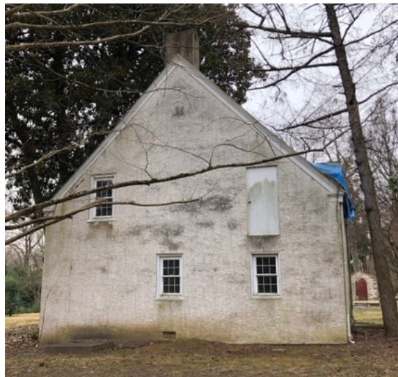
Fig. 39. The east face of the servants quarters as built, although one window was later altered by Upper Merion Township to create an emergency exit in the 1970s. The stairs that led from the door to the ground have since been removed. Current photo.
