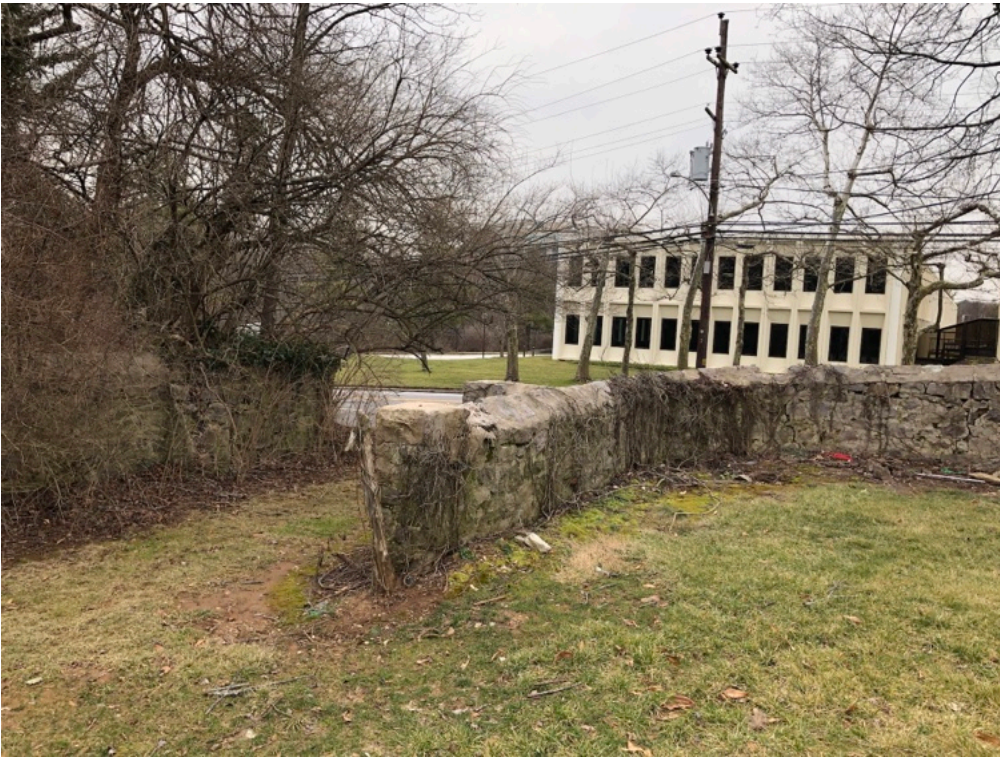
Fig. 29. Walls at the old entrance to the property on Moore Road, looking west. Current photo.
