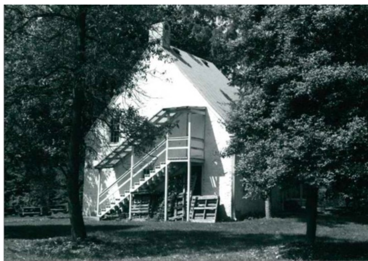
Fig. 45. The east side of the house, showing the emergency exit and stairs (since removed) from the servants quarters second floor. Photo by Dave Broida in 1979.
