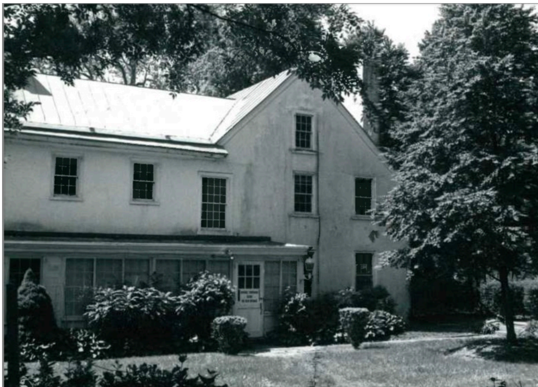
Fig. 12. The north side of the house showing the enclosed porch (since removed.). Photo by Dave Broida in 1979.
