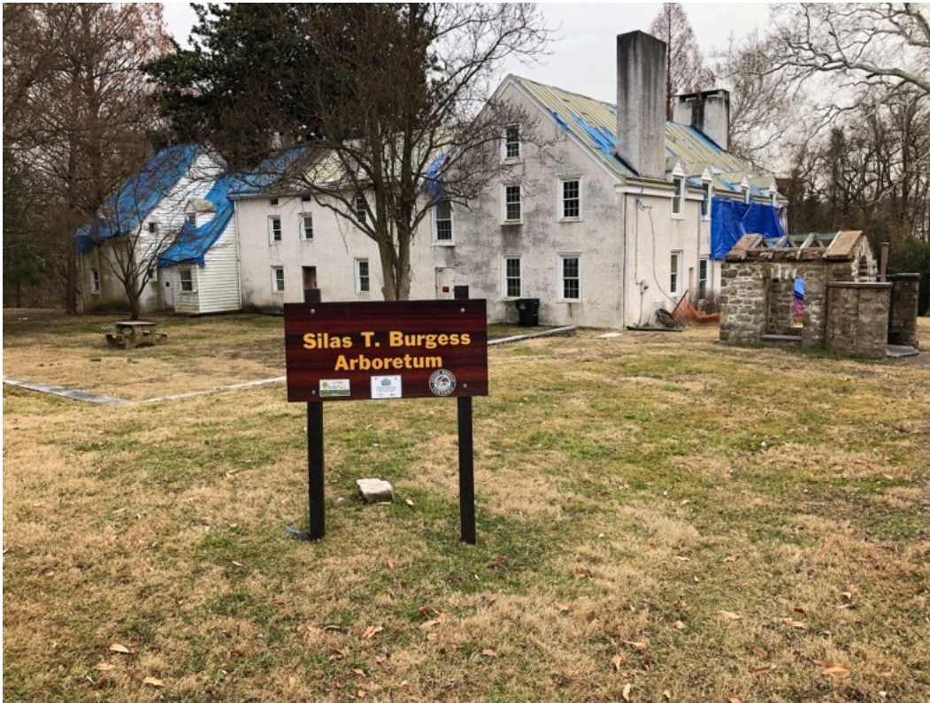
Fig. 15. The north and west side of the house, looking southeast. On the right is the Okie addition with dormer windows that break the roofline and cross-gabled roofline. The large chimneys are also visible. Current photo.
