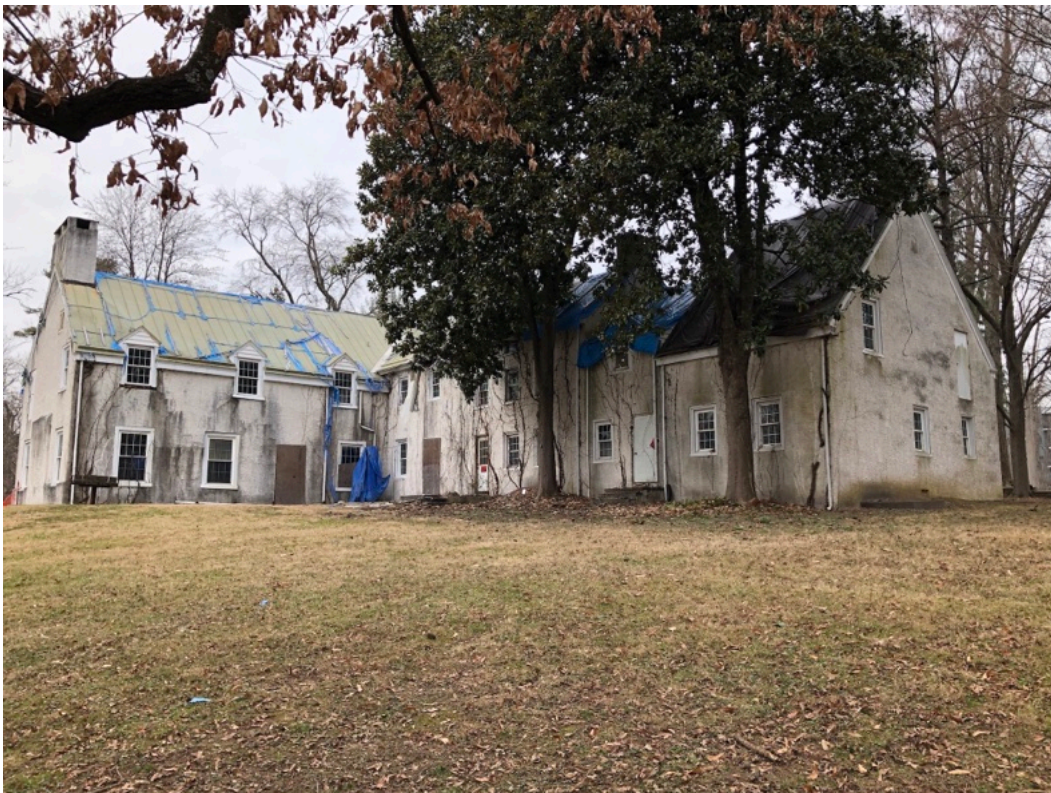
Fig. 16. The south and east side of the house, looking northwest. On the left is the Okie addition with dormer windows that break the roofline. Current photo.
