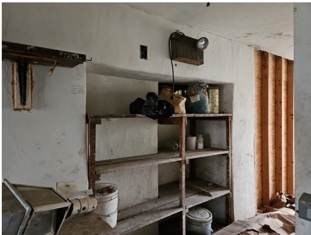
Fig. 16. The fireplace wall, viewed from east side, that is, from the proposed location of the log structure. From the archive of the King of Prussia Historical Society.
