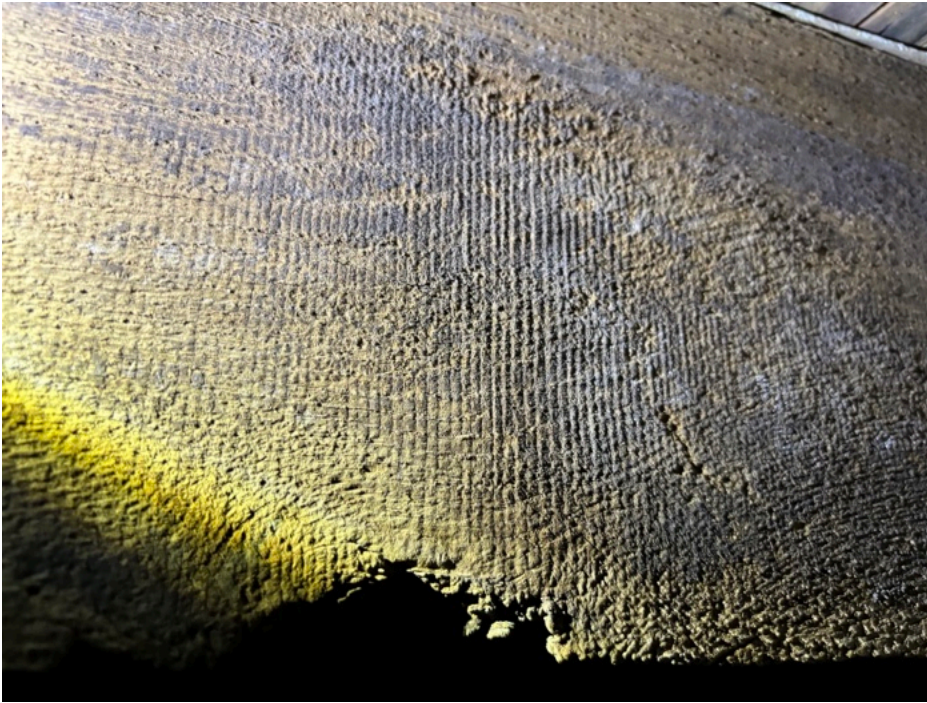
Fig. 23. Joist under the circa 1810 stone addition showing vertical, evenly spaced saw marks. From the archive of the King of Prussia Historical Society.
