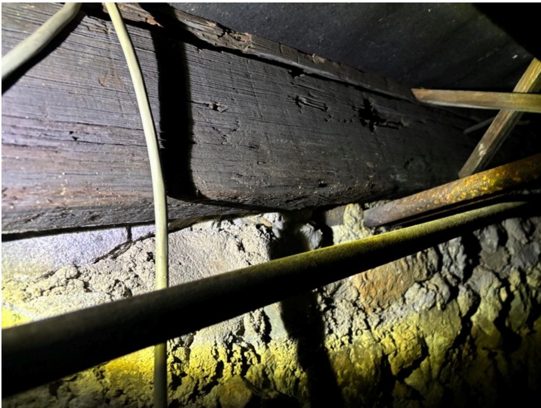
Fig. 30. Joist under the house east of the circa 1810 addition, showing marks not indicative of machine sawing. From the archive of the King of Prussia Historical Society.
