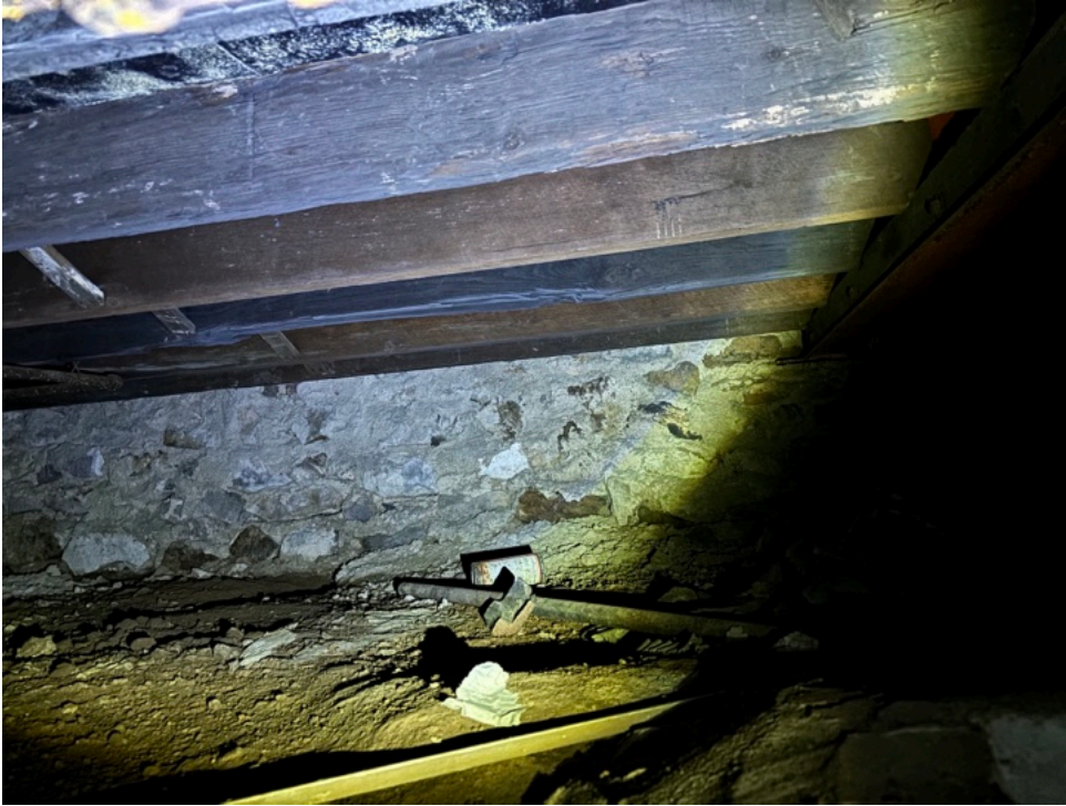
Fig. 27. Joist under the house, east of the circa 1810 addition, showing different colors of wood. From the archive of the King of Prussia Historical Society.
