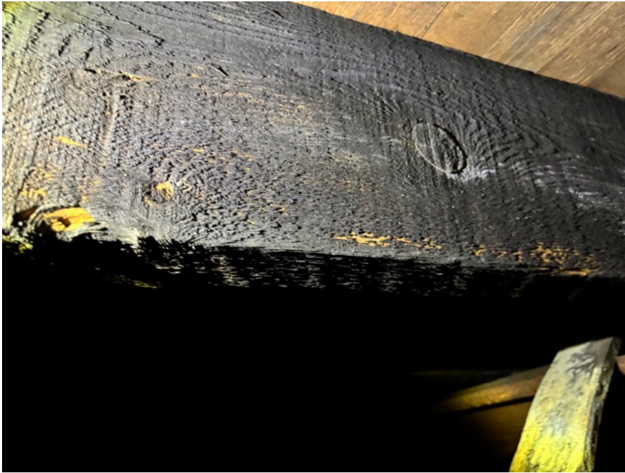
Fig. 25. Joist under the circa 1820 addition showing vertical, evenly spaced saw marks. From the archive of the King of Prussia Historical Society.
