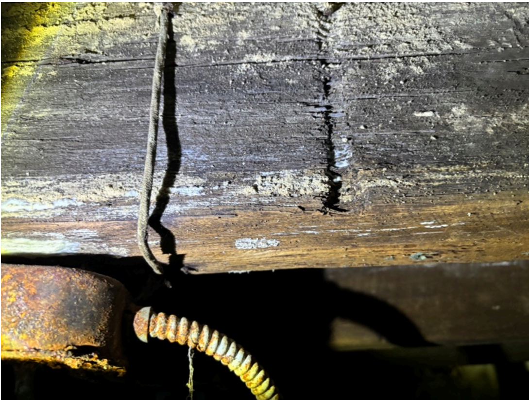
Fig. 34. Joist under the house east of the circa 1810 addition, showing marks not indicative of machine sawing. From the archive of the King of Prussia Historical Society.
