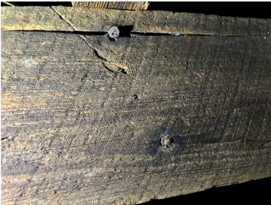
Fig. 26. Support beam under some of the joists in the circa 1820 addition showing curved saw marks. From the archive of the King of Prussia Historical Society.
