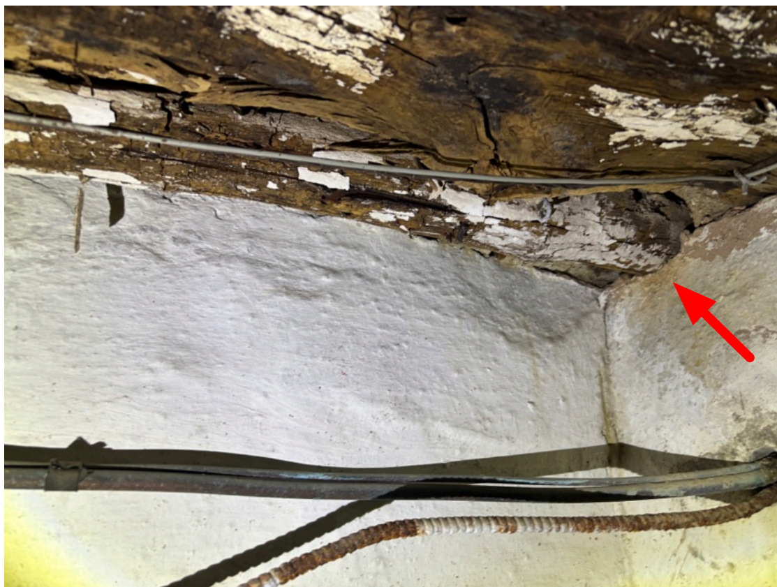
Fig. 18. An opening in the fireplace wall in the basement, showing rough wood, one piece of which is cylindrical in shape. From the archive of the King of Prussia Historical Society.
